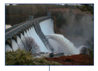
This picture shows water being released under pressure, after it has turned the turbines inside the dam to generate electricity (Laggan Dam). Photo courtesy of Roy Dyckhoff
